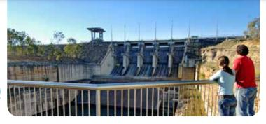
The Wivenhoe Dam was built on the Brisbane River after the 1974 flood event. The dam wall is 2.3 kilometres long, with five radial gates to release water. While its primary function is to provide safe, reliable water supply, the dam also provides flood mitigation.
